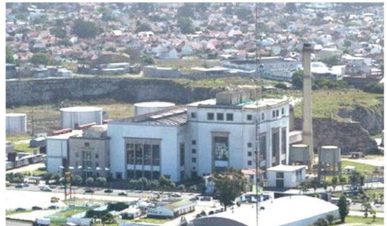
thermoelectric plant built in 1950
