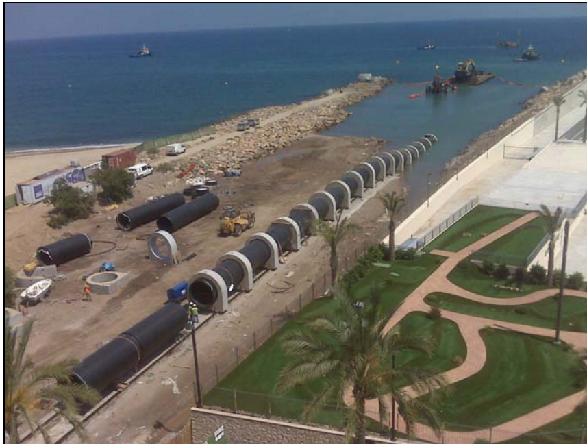
Figure 11 Aguilas: the pipe, during launching at the shore.
