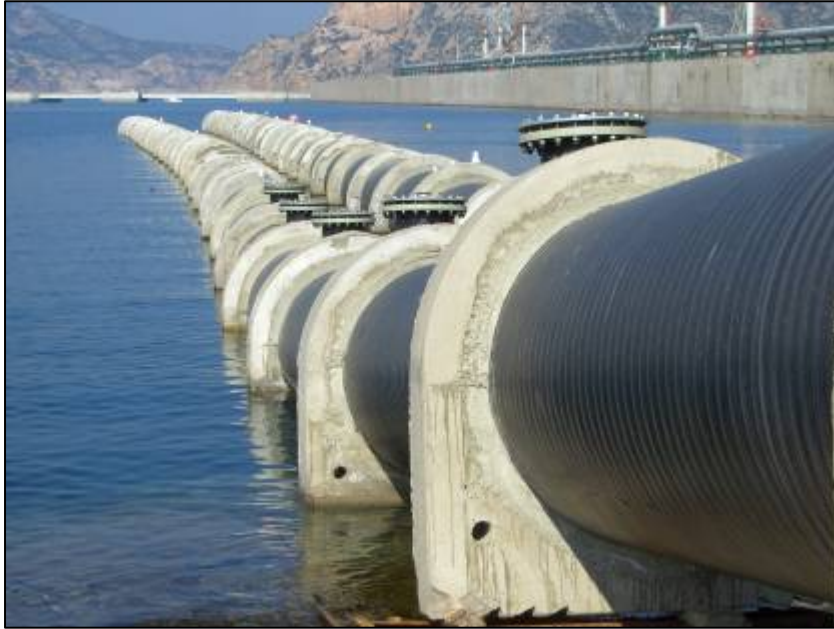
Figure 8 : Valdelentisco pipes during launching
