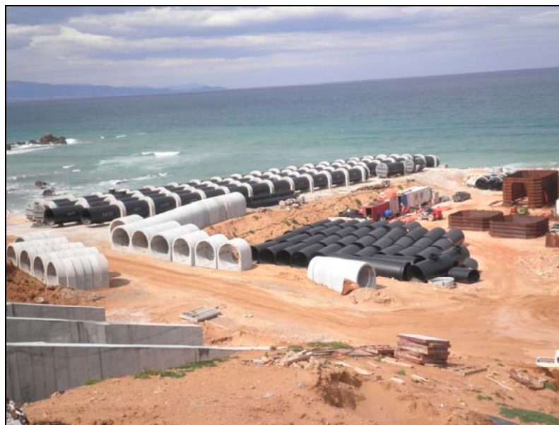
Figure 7 Works on land at Koudiet.
