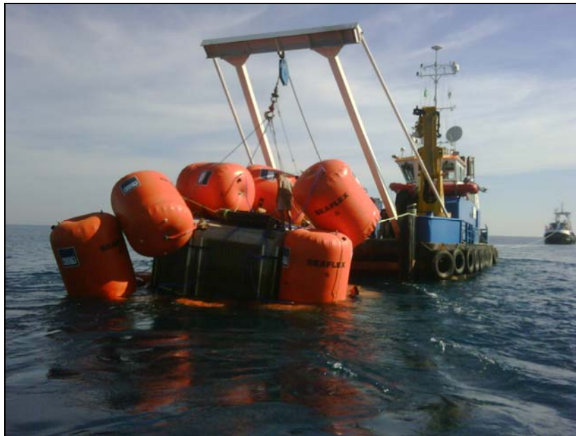
Figure 10 Cap Djinet: intake tower.
