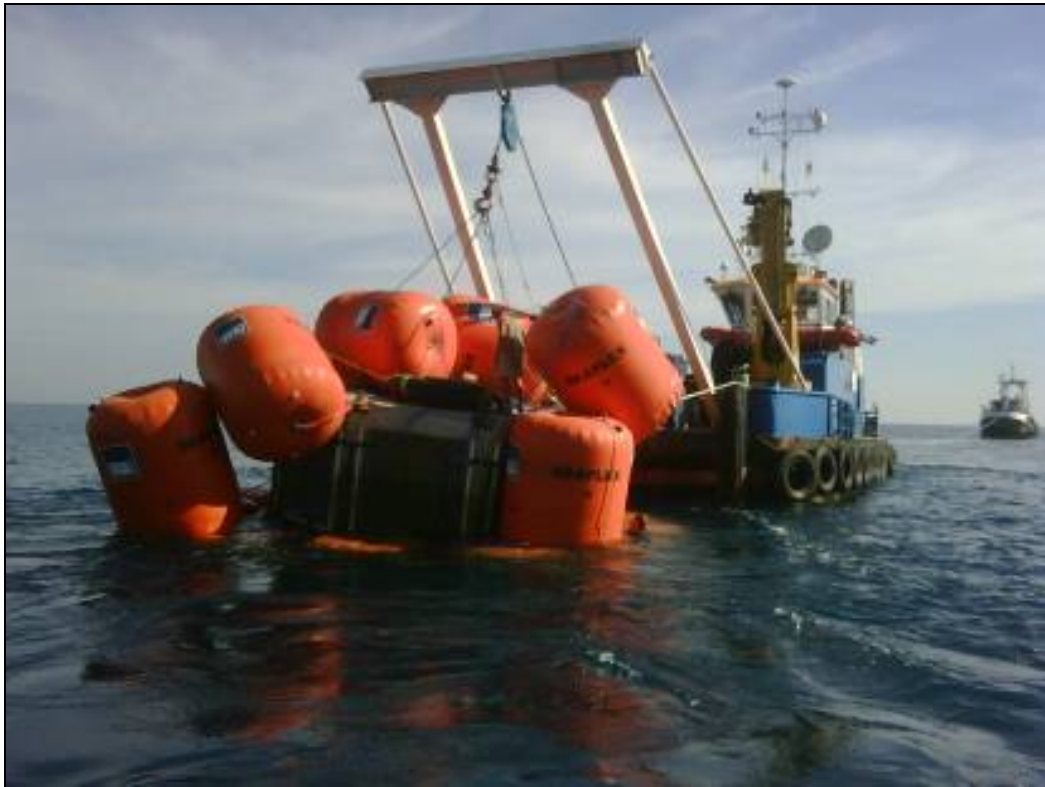
Figure 10 Cap Djinet: intake tower.
