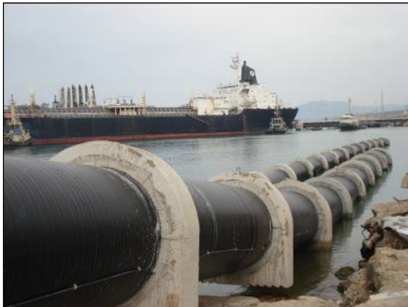
Figure 9 Skikda: pipes during launching at the port
