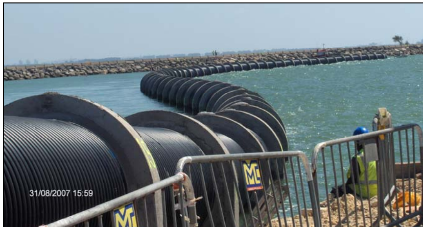
Figure 3. Cadiz outfall of 1800 mm, during sinking
