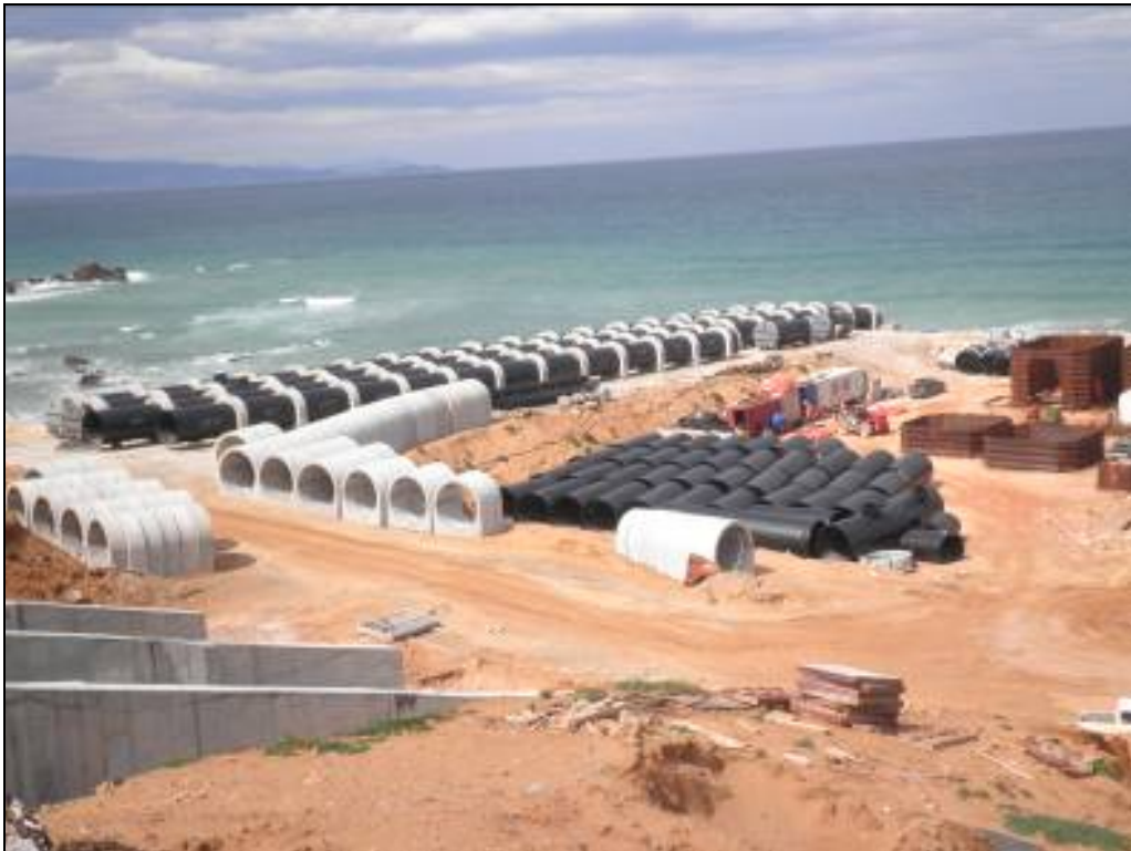
Figure 7 Works on land at Koudiet.
