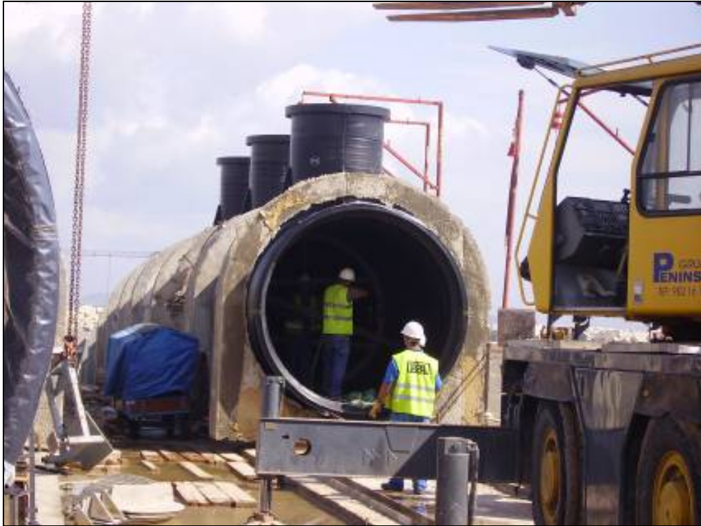
Figure 4 Algeciras outfall (diffuser zone), during ballasting
