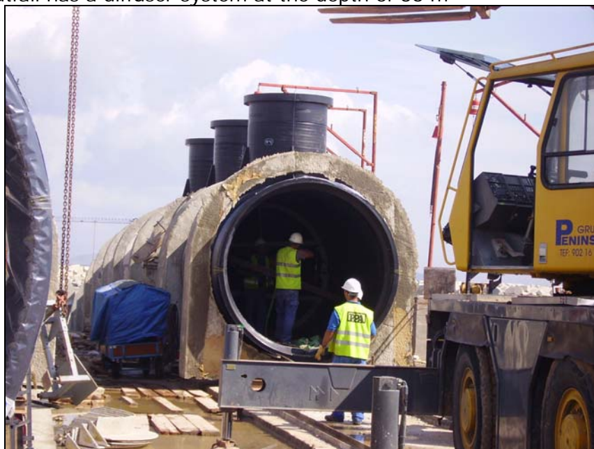
Figure 4 Algeciras outfall (diffuser zone), during ballasting
