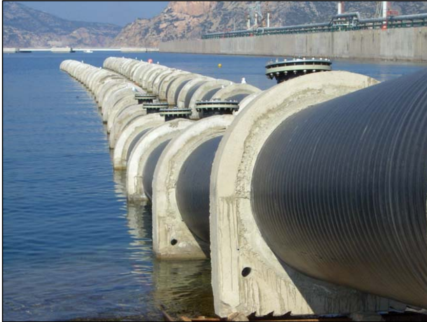
Figure 8 : Valdelentisco pipes during launching
