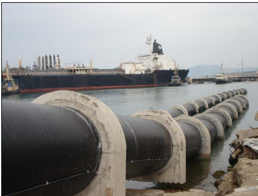
Figure 9 Skikda: pipes during launching at the port
