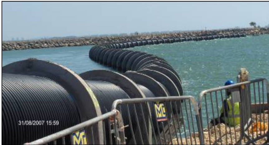
Figure 3. Cadiz outfall of 1800 mm, during sinking
