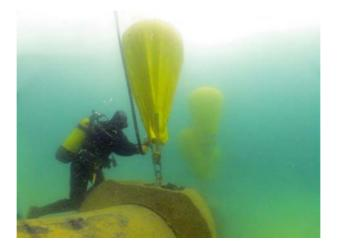
Last case is the connexion of pipes segments with diameter between 710 and 1600 wich are less complicated to sink. Here the connections between segments can be done on the same day using long studs to joint the flanges together.
