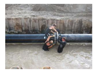
For large diameter pipes (from DN 1600) and long segments with complicated sinking manouvers, the best option is to execute the sinking in such a way that the head of the new sunken segment lies on the seabed in paralel to the head of the already laid pipe. This will allow for easy removal of the blind flange plates assemblies. Then, divers will lift the two heads with lifting bags and proceed with the final bolting of the flanges.
