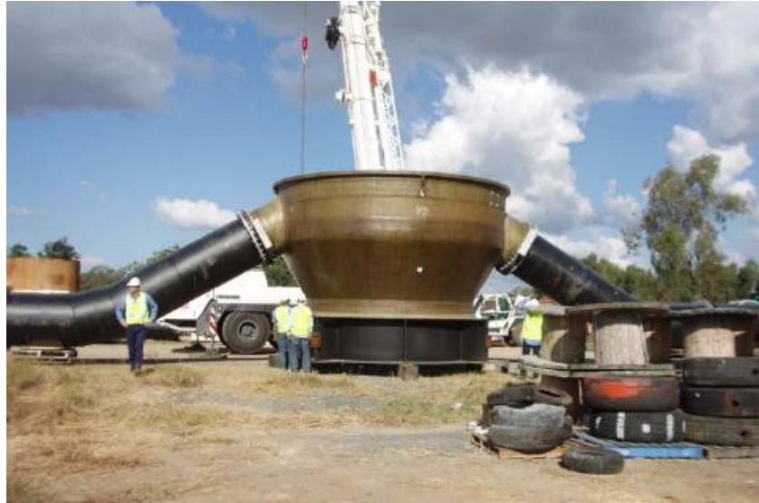
Figure 1. ‘Diffuser head’ and ‘arms’ prior to installation on seabed
