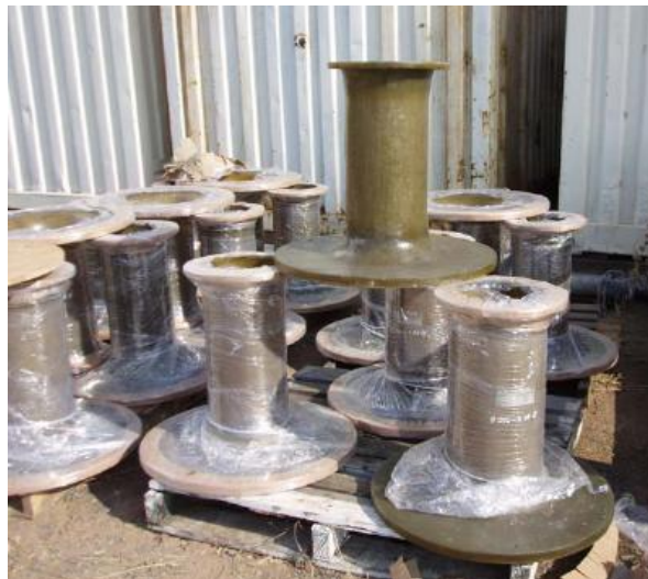
Figure 2. GRP flanged nozzles prior to installation
