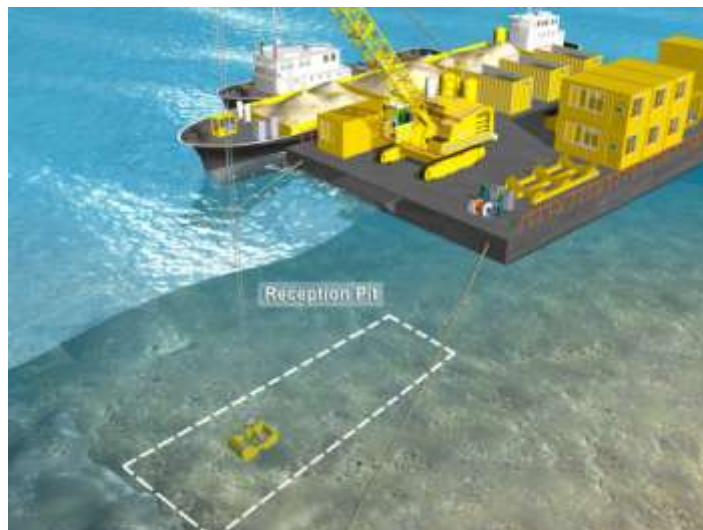
Picture 2: Excavating the reception pit
