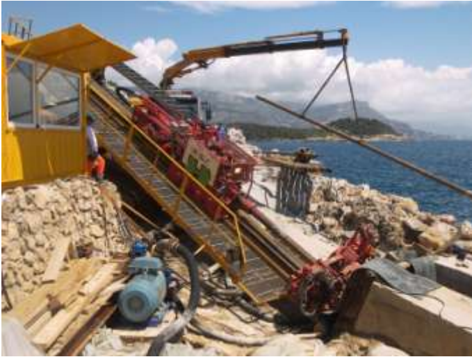
Picture 6a Drilling from onshore
