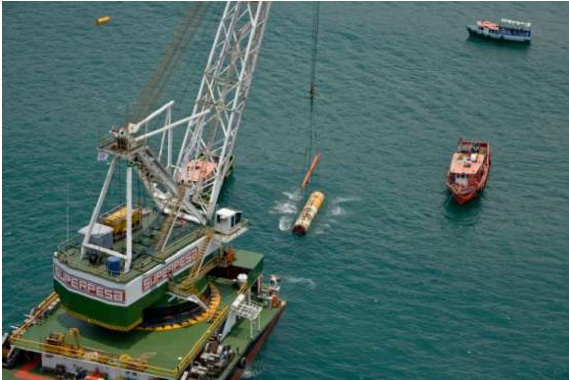
Picture 3: Recovery by crane
