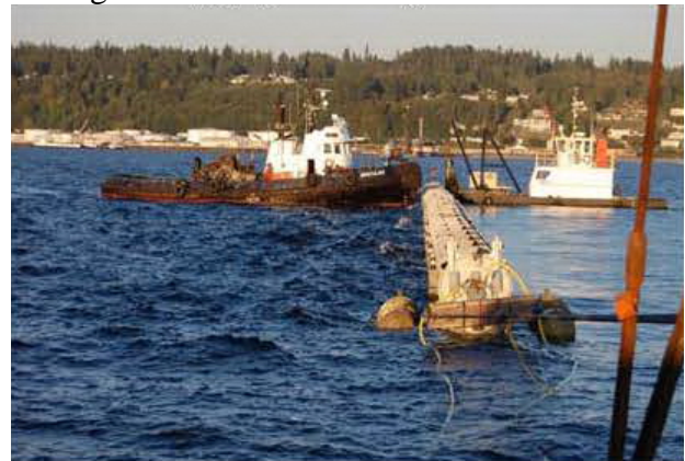
Figure R – Pulling barge in center kept on line and at proper tension by the twin tugs in the upper left. Remaining boats used to keep pipe on alignment.
