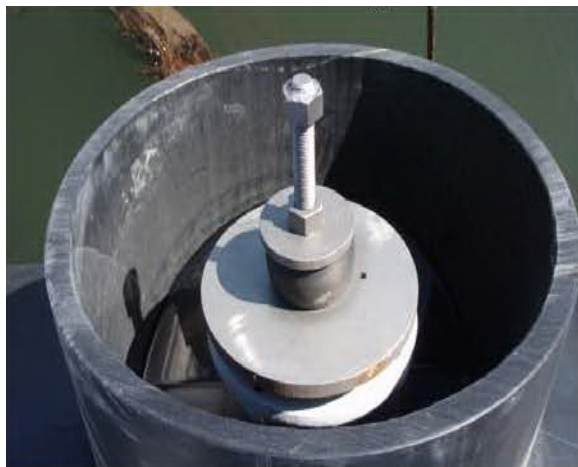
Figure H – Diffuser and cap with surrounding HDPE shroud.
