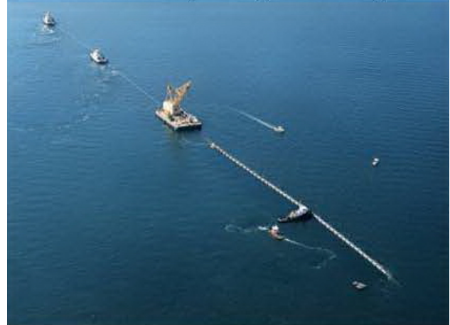
Figure R – Pulling barge in center kept on line and at proper tension by the twin tugs in the upper left. Remaining boats used to keep pipe on alignment.
