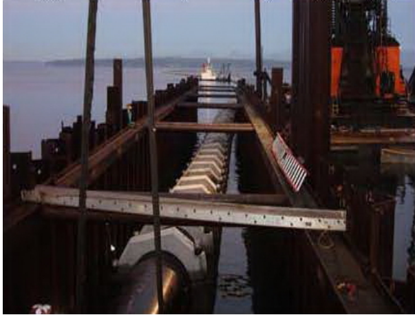
Figure Q – South HDPE outfall pipe as it is pulled into the shoring for attachment to the wye and start of controlled submergence
