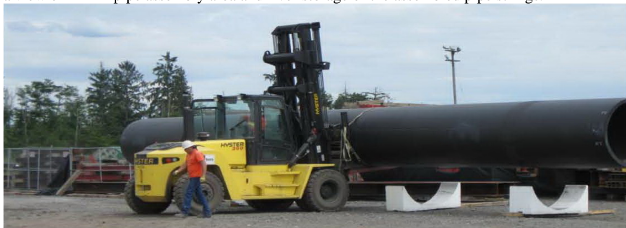
Figure K – 63" diameter by 60 foot long HDPE sections being moved around the assembly yard.
