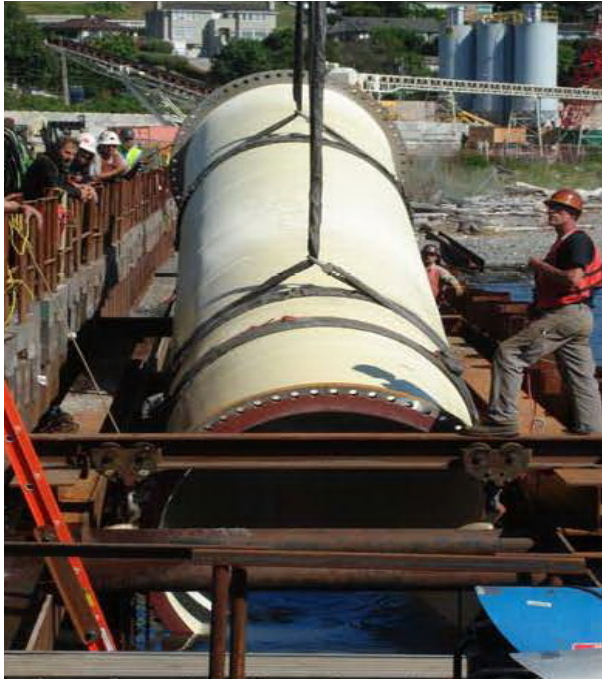
Figure A – 84” flanged steel pipe section being installed in the shored trench.
