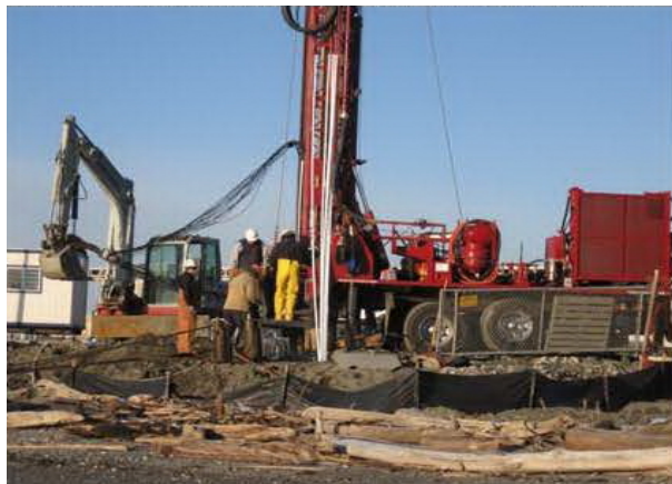
Figure U – Anode well drilling and anode placement.
