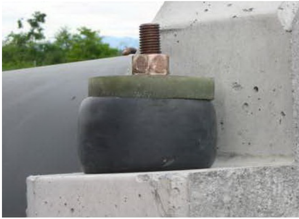
Figure E – Anchor bolt, rubber compensator block, FRP washer and nut after tensioning.
