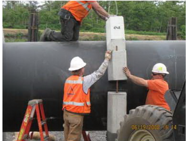
Figure M – Attaching concrete collars
