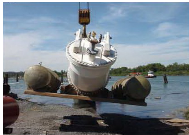
Figure I – End gate structure as the pipe is placed into the river.
