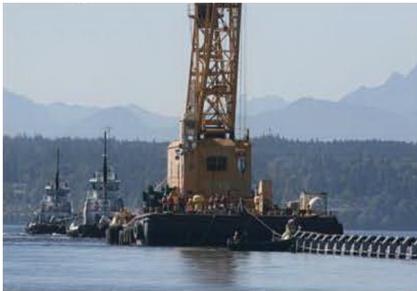
Figure S – On the water view of the outfall pipe, pulling barge and tugs.
