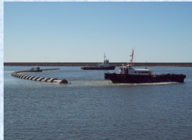
Installation of Mar del Plata outfall
